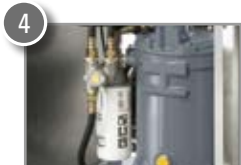
4 Oil separator & oil filter
