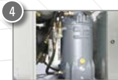
4 Oil separator & oil filter
